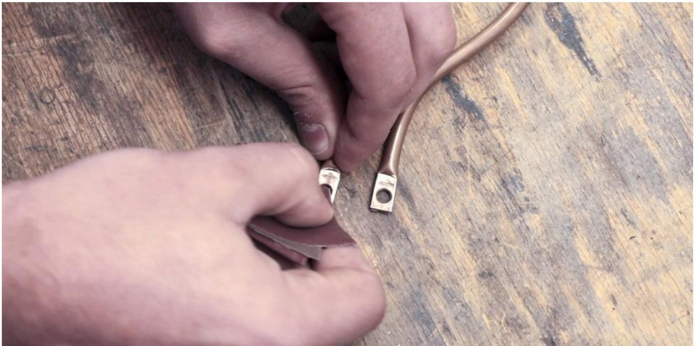
Fig. 51: Sanding contact surfaces
